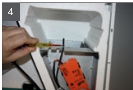
Installation position of temperature sensor 3
