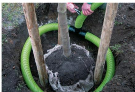
An additional pipe section provides the connection between the loop and the surface.
