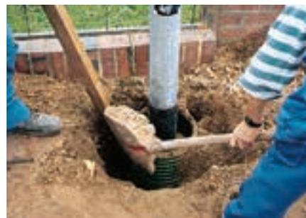
Then, backfill and compact the remaining gap around Furowell with native non-cohesive soil and provide a cover layer.
