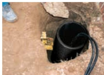
Then, fill the annular space in the pole foundation conduit with sand. Backfill the upper area of the annular space with tamped concrete for lateral adjustment and to prevent water ingress.
