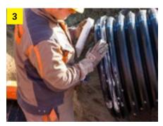
Keep the pipe, the sealing ring and the coupling clean. Then apply a sufficient amount of lubricant to the sealing ring and coupling. Make sure that the sealing area is free of dirt. Deepen the embedding in the area of the couplings as required. In order to prevent the profile sealing ring from resting on the bearing, the pipe end to be installed can rest on square timber.
