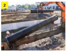
Move the sedimentation pipe to the installation position using lifting equipment. The crown marking must face upwards! The integrated flow separator faces downwards!
