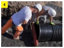
Use a long lever to install the pipe. Place a board or square timber under the unattached pipe end to prevent damage to the pipe. Pipes must be installed horizontally. Mark the insertion depth on the pipe beforehand. Afterwards, create the pipe gradient by aligning the pipe. When completing the lower embedding by means of tamping, make sure that the bottom side of the pipes rests completely on the compacted foundation.
