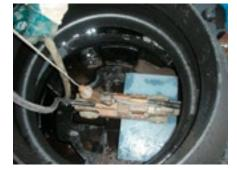
Inspection of flushing results with pan and tilt camera, camera on the maintenance console in the start shaft of a SediPipe level system
