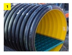
Mount profile sealing rings into the first corrugation trough on each side while still outside the excavation pit. The pipe must be clean.
