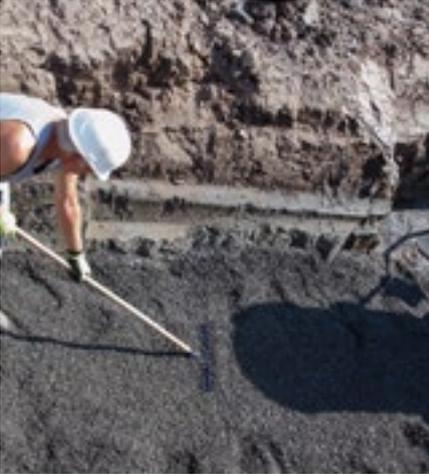
In addition to the regulations of DIN EN 1610, observe the specifications of DIN 18300 "Earthworks" (*Erdarbeiten*) in the latest version regarding excavating the pit and creating the lower embedding for SediPipe level.
