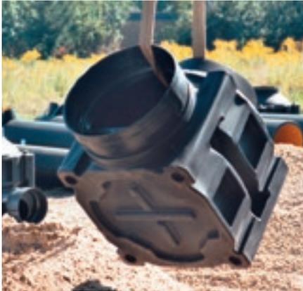
Transport using appropriate hoisting slings
