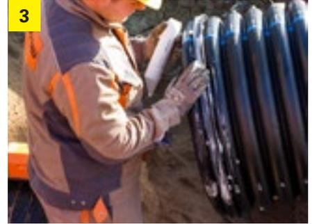
3 Keep the pipe, the sealing ring and the coupling clean. Then apply a sufficient amount of lubricant to the sealing ring and coupling. Make sure that the sealing area is free of dirt. Deepen the embedding in the area of the couplings as required. In order to prevent the profile sealing ring from resting on the bearing, the pipe end to be installed can rest on square timber.
