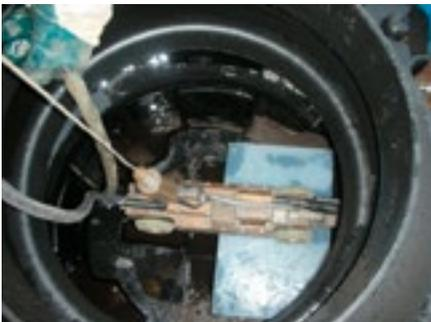
Inspection of flushing results with pan and tilt camera, camera on the maintenance console in the start shaft of a SediPipe level system
