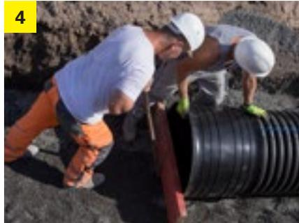
4 Use a long lever to install the pipe. Place a board or square timber under the unattached pipe end to prevent damage to the pipe. Pipes must be installed horizontally. Mark the insertion depth on the pipe beforehand. Afterwards, create the pipe gradient by aligning the pipe. When completing the lower embedding by means of tamping, make sure that the bottom side of the pipes rests completely on the compacted foundation.
