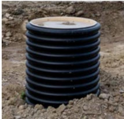
Extension pipe with temporary construction site cover
