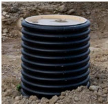
Temporary construction site cover for extension pipes
