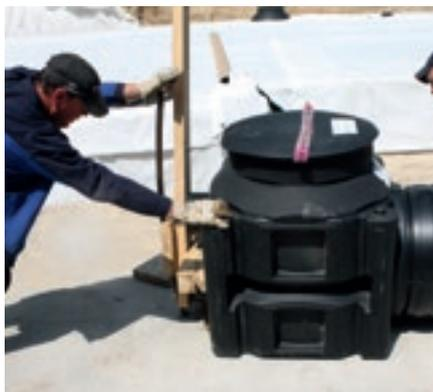
Place the second shaft at the appropriate height on the prepared planum. Afterwards, prepare the coupling connection and mount the shaft onto the sedimentation pipe. Connect supply pipe and drainage pipe according to design specifications (see Section 4.5).
