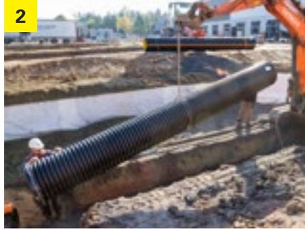
2 Move the sedimentation pipe to the installation position using lifting equipment. The crown marking must face upwards! The integrated flow separator faces downwards!
