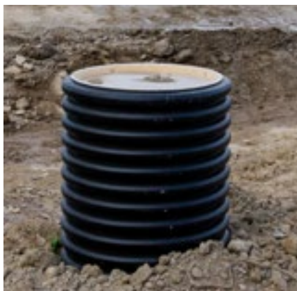
Extension pipe with temporary construction site cover
