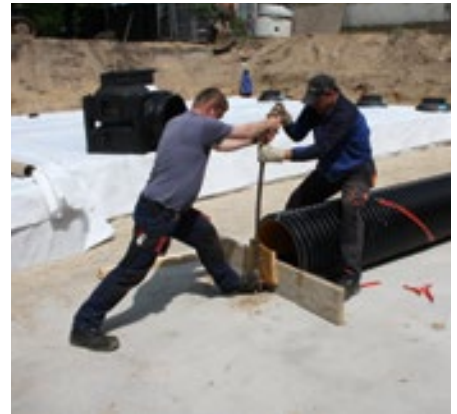
Installation of sedimentation pipe
