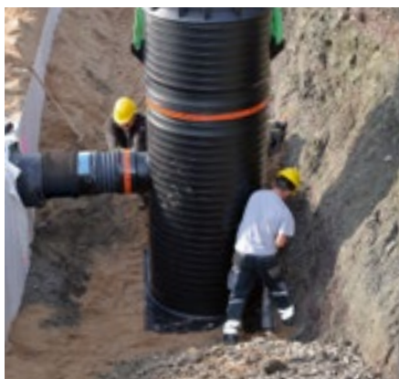
Example: target shaft with Rigofill storage/infiltration system
