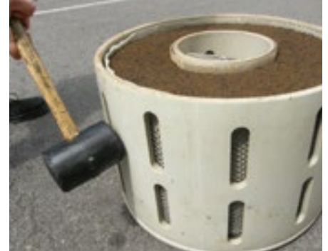
Compacting the substrate
