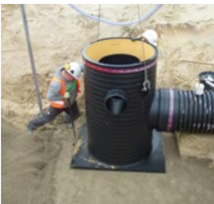
Installation of target shaft
