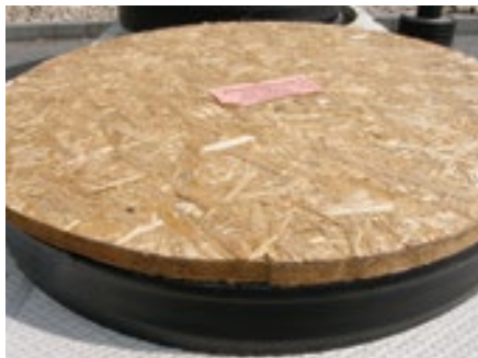
Protective cover for shaft with concrete cover
