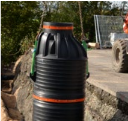
Transport using appropriate hoisting slings
