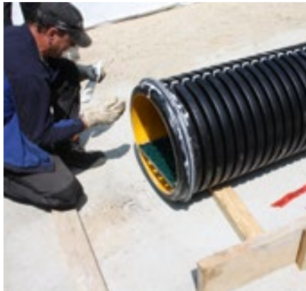
Sealing ring with lubricant
