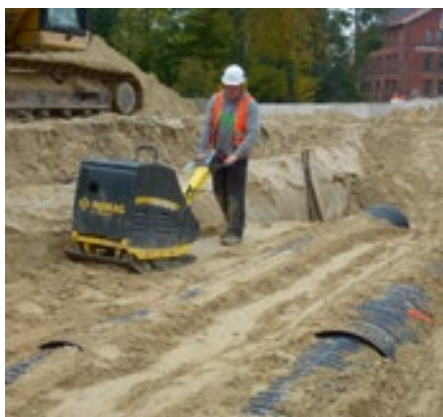
Compacting of lateral backfilling
