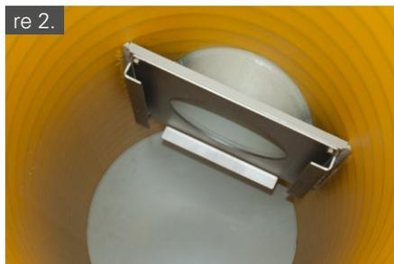
3. After that, insert the valve through the shaft opening and with the square base plate made of dark PE-HD into the stainless steel channel of the branching pipe connection. The valve will slide down the channel to the lower arrester thanks to its own weight and without canting. The handles of the lifting bar are then positioned right under the shaft opening at the same height as the fixture.
