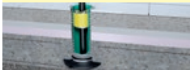
Foundation slab lead-through for buildings without basements
