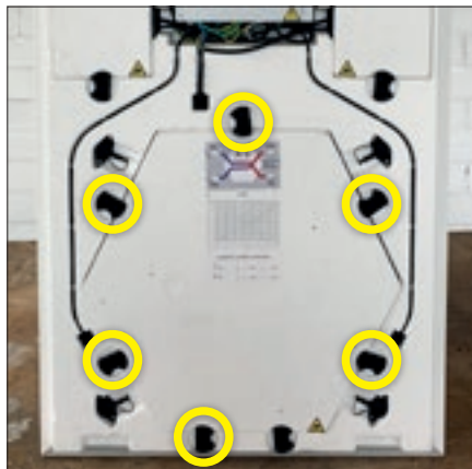
Position of the heat exchanger interlocks
