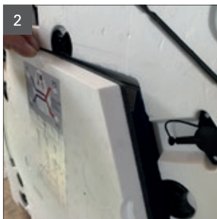
Remove the EPS cover of the heat exchanger.
