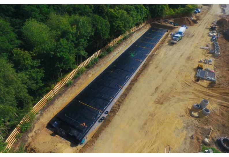
RigoCollect® stormwater retention with SediPipe® XL 600/12 as a pretreatment system
