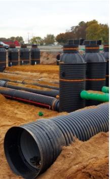
The DIBt-approved systems SediSubstrator and Rigofill inspect will now treat, store and subsequently infiltrate the surface water of the Nievenheim-Ost filling and service area in a controlled way. The underground infiltration system with sedimentation path by FRÄNKISCHE thus protects the groundwater along the A57 motorway, one of the arterial roads along the Lower Rhine, with high treatment performance and little space requirements.
