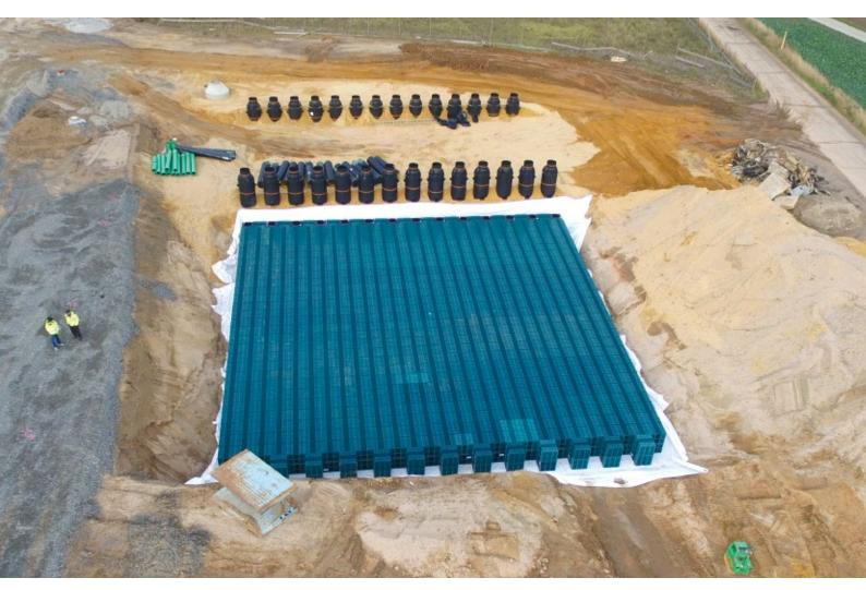
Stormwater treatment with subsequent infiltration
